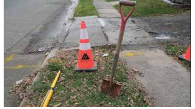
12 RAHWAY IS AT WORK Behind-the-scenes: The City at work
